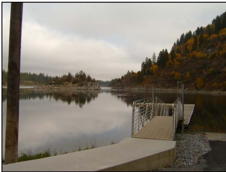
NORTHPORT LAUNCH LOOKING UPSTREAM.
